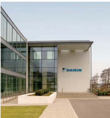
Daikin Airconditioning UK Ltd, Weybridge Head Office
